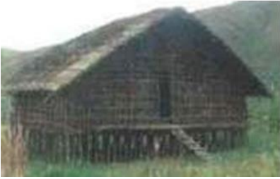
Figure 40. 'House of one thousand legs', low type of house in the Bird's Head area, also used as a wuon educational institution compound.
