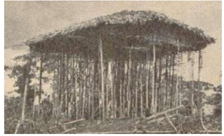
Figure 41. Mbol qalit 'house of one thousand legs' tree top type house in the Bird's Head area, also used as a wuon educational institution compound.
